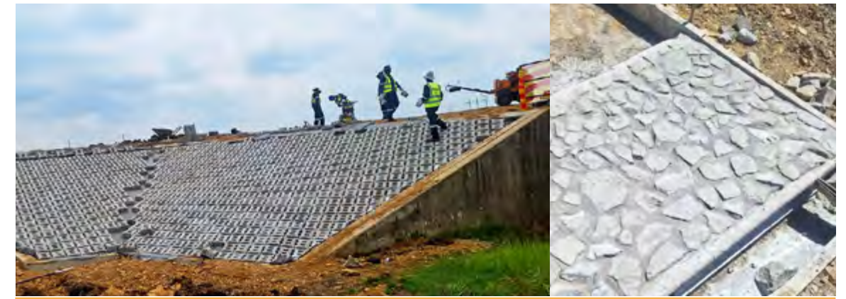
7 Civil & structural engineering of the Matla Washaway, Mpumalanga, SA | Sasol Gas
