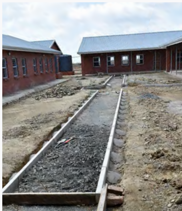
Themba Mzizi Primary School | DPW Eastern Cape
