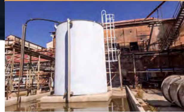
Structural engineering: mine water tank support & bund, Mpumalanga | Evander Gold Mine
