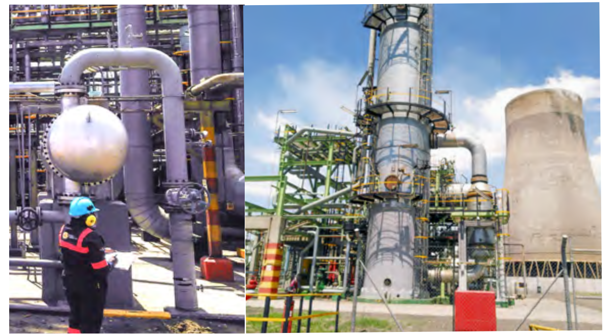
7 Inspection of various structures within the Sasol Secunda Plant, Secunda, SA | Sasol Secunda Operations
