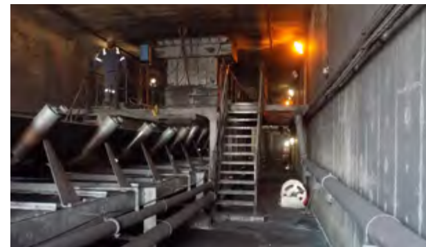
Structural inspection inside Syerfontein Mine, Secunda | Sasol Mining
