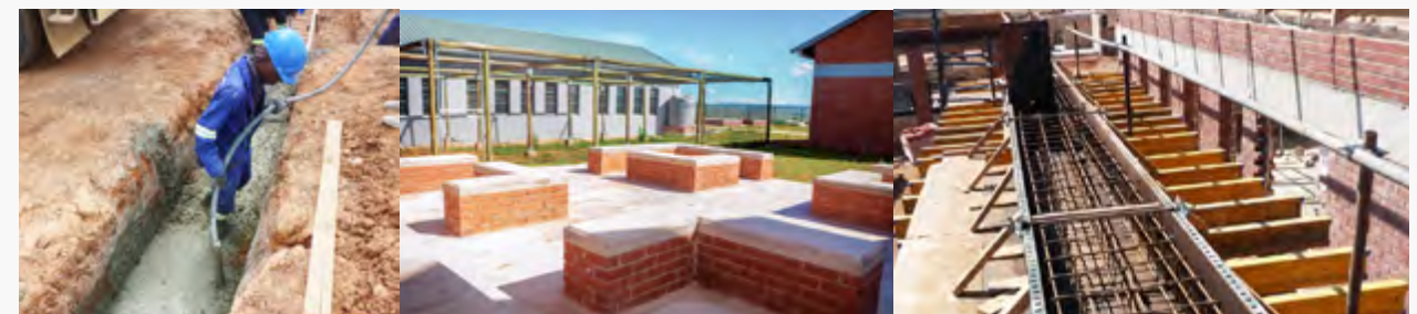
MegaSchools Project. Structural Engineering for Pongseong Junior Secondary School. Pongseong Village Matatiele, Eastern Cape | COEGA CDC
