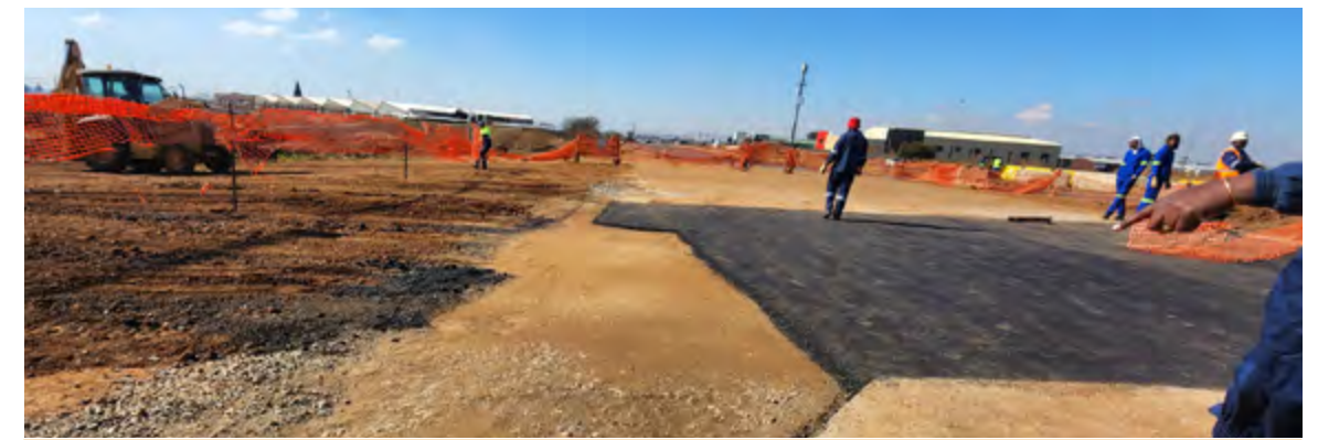
7 Project management of SAP road construction, South Africa | Sasol Gas
